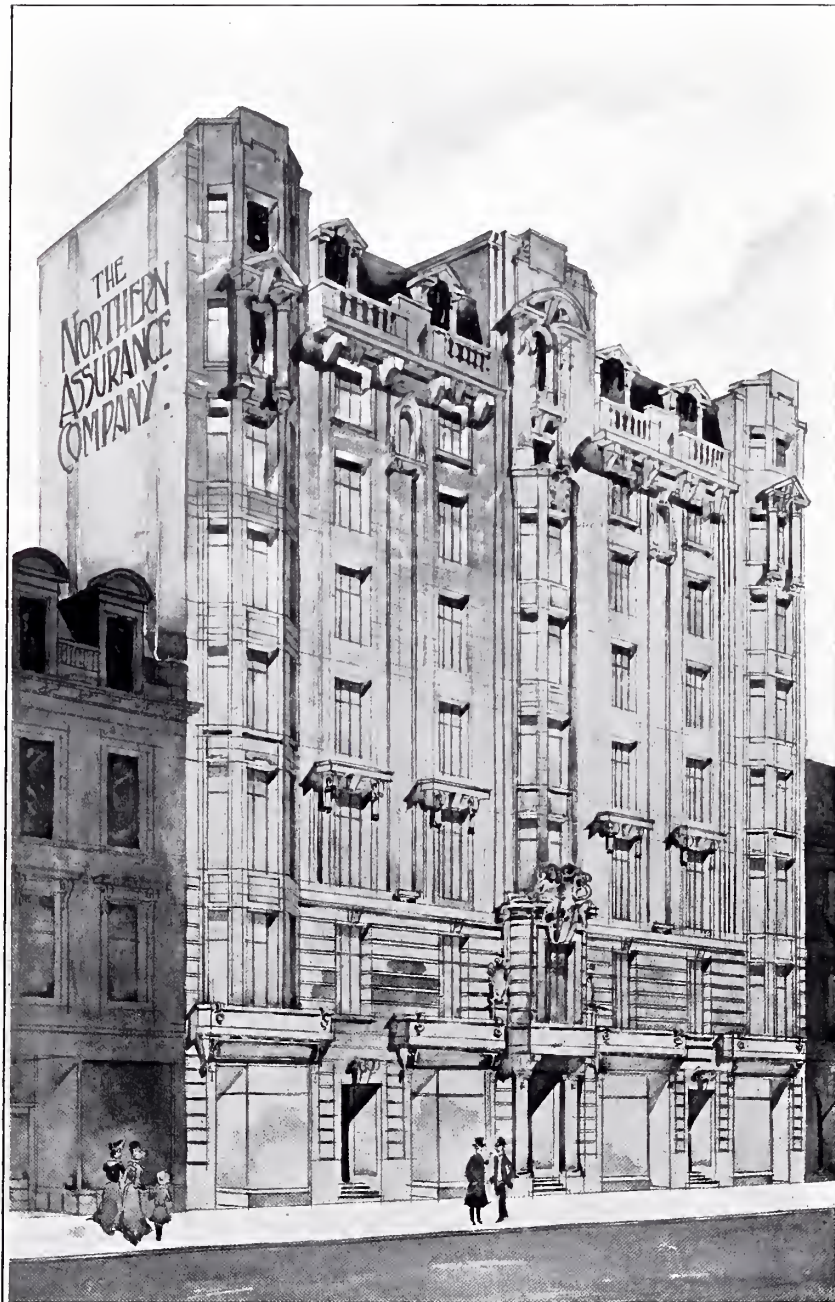
683. Northern Assurance Company's Buildings, St. Vincent Street, Glasgow, JOHN A. CAMPBELL, Architect. Masonry: P. and W. Anderson, Ltd., 64 Douglas Street, Glasgow.
